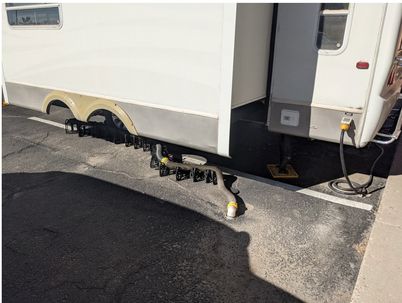
Code compliant water hook-up (September 16, 2021)
